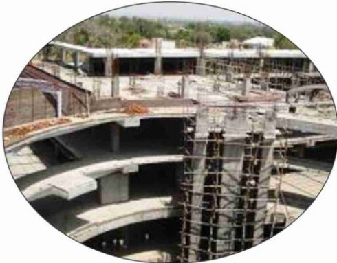
PT SLAB IN MALL
