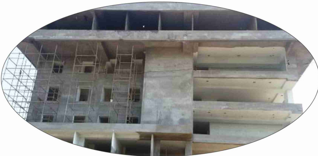
PT SLAB & BEAM FOR LARGE CANTILEVER
