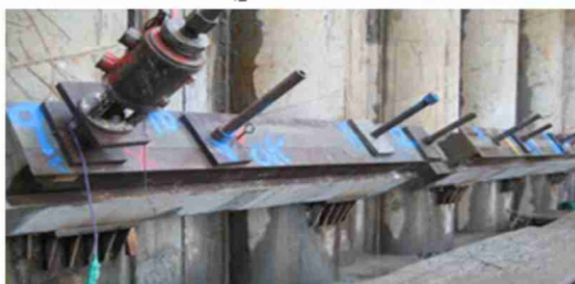
INCLINED ANCHOR FOR BASEMENT EXCAVATION
