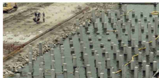
VERTICAL ANCHOR FOR FOUNDATION
